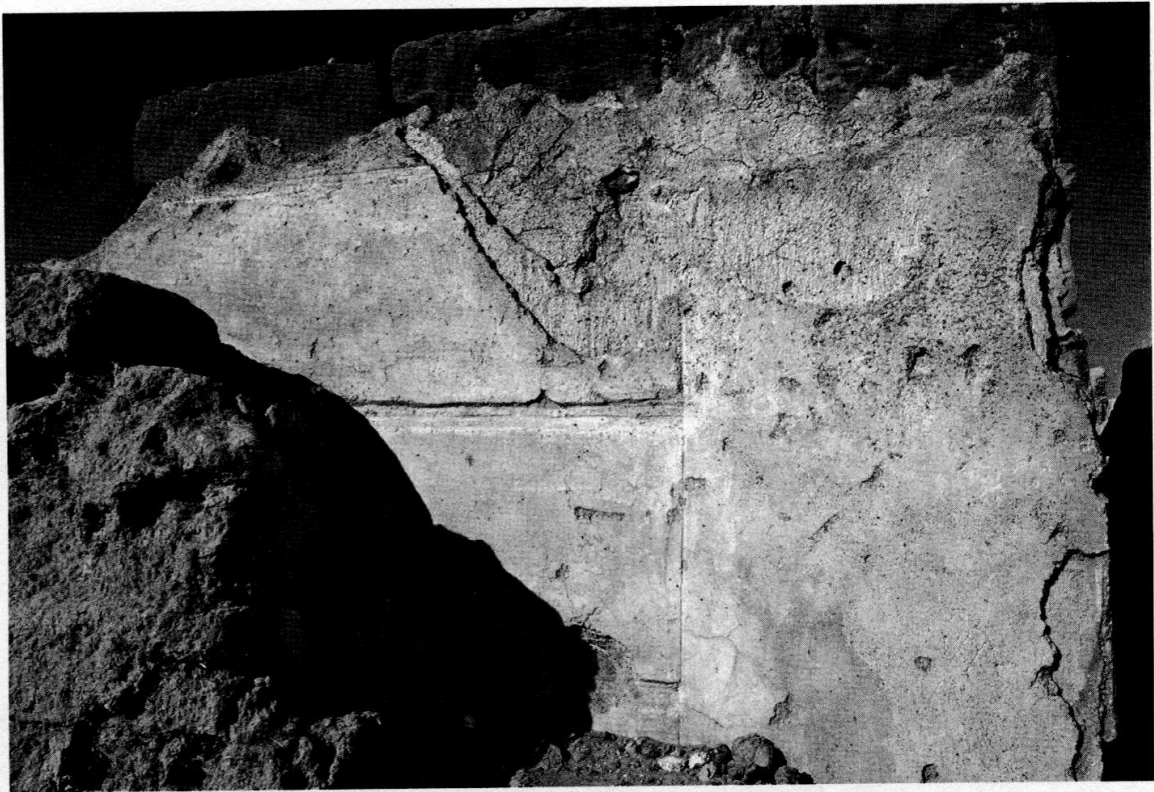
Fig. 22. Detail of the plaster on the original façade of temple ST 18.
